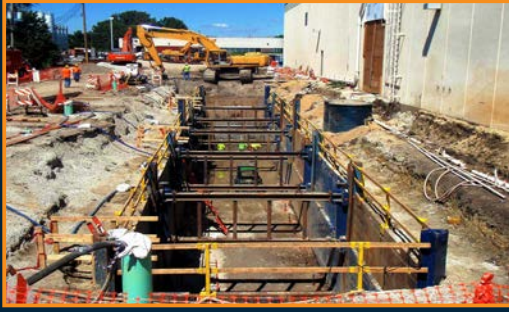
Slide Rail Shoring
